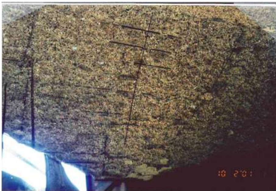
Fig.1.1: Fire Damaged Slab
